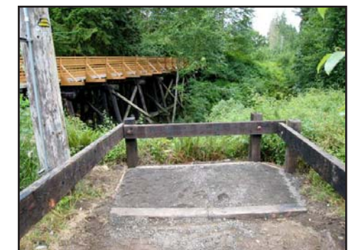
New overlook at the newly finished RR trestle
